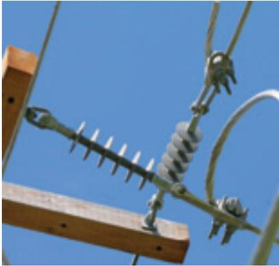
**SILICONE COMPOSITE INSULATORS** combine the technologies of a fiberglass reinforced rod, metal fittings and our extensive knowledge of elastomeric insulation to produce a high quality composite insulator. Since 1980, thousands of Silicone Insulators have been installed by utilities worldwide in a variety of environments. Continued outstanding performance is proof of their superior quality and design.
