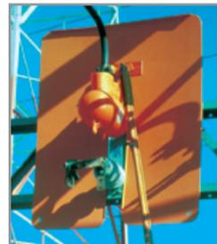
Barrier and Switch Jaw Guard installed on a Substation Switch.
